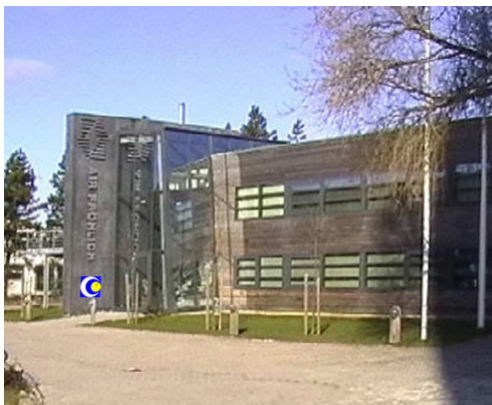
Metrologic office building in Horsholm
